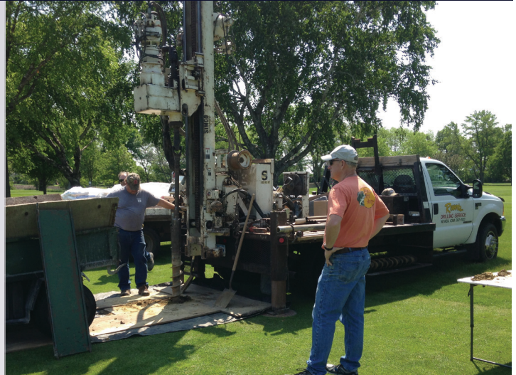
Dr. Keith Schilling, University of Iowa Research Scientist and Engineer, supervises the drilling of one of the six test wells used in the Water Quality Research Project.
